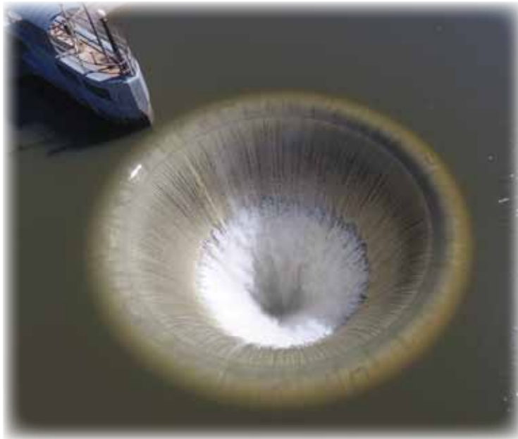
The ring gate at Owyhee Reservoir, also known as "the glory hole" spills water on April 3. According to the Owyhee Irrigation District, this spring was the first time the ring gate spilled water since 2011. Owyhee Dam is located in Malheur County, Oregon and at the time of construction (1932) was the tallest dam of its type in the world at 417 feet. The reservoir stores more than 1.2 million acre-feet of water that is used to irrigate 120,000 acres of farm land in Oregon and Idaho.
