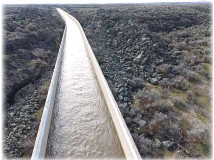
The Idaho Department of Water Resources is working with canal companies to run excess water into the ground to recharge the Snake River Plain Aquifer.
