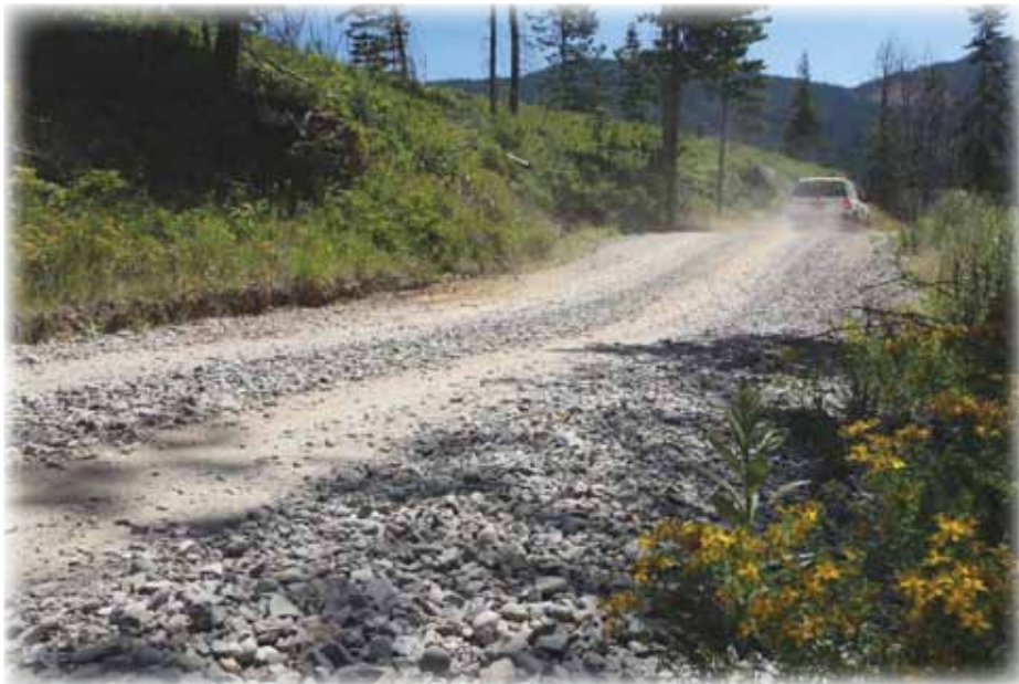
Rolling dips are an alternative to cross drain culverts. Photo Courtesy Robert Barkley, Idaho Department of Lands
