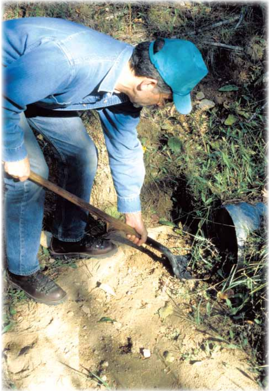
Keeping culverts open after a forest fire is critical.
