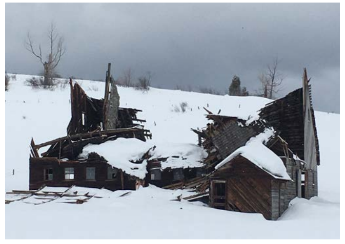
These pictures show a barn in Bear Lake County before and after it collapsed this winter under the tremendous weight of snow and ice. Photos by Jim Parker
